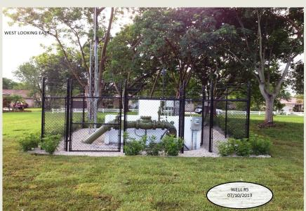
Here, is a picture of a rehabilitated well that was just competed in July. The scope of the project included evaluating the current well condition, redesigning the exposed piping to meet County requirements, increasing the flow capacity of the well to approximately 250 gallons per minute over the existing flow capacity, and other items. To close out the project we installed high-grade security fencing and new landscaping.
